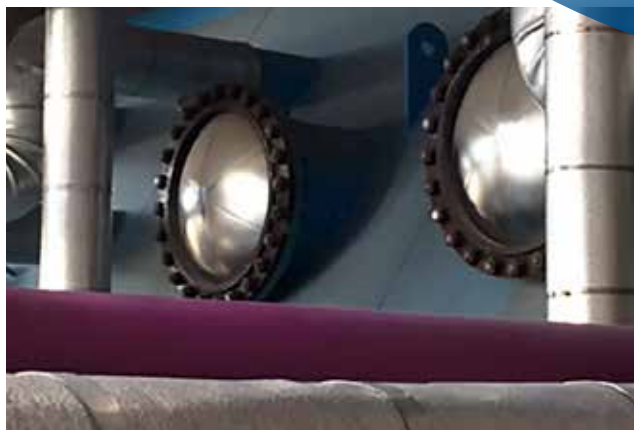
DV(F)-FB-G Rupture Disk providing overpressure relief for a steam surface condenser
